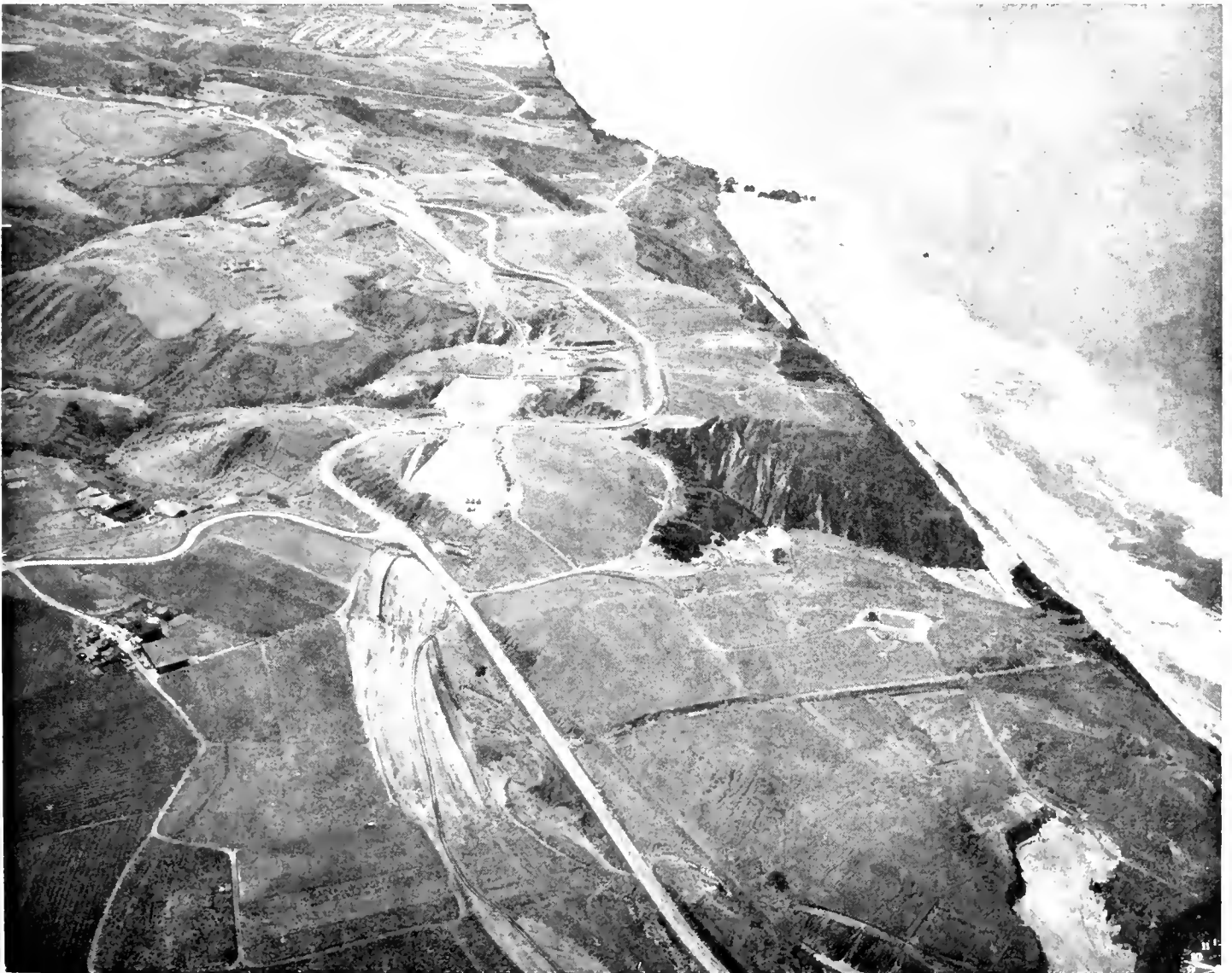
View showing progress of grading operations for Skyline Boulevard from Edgemar Road to junction of Routes 55 and 56 in Daly City
